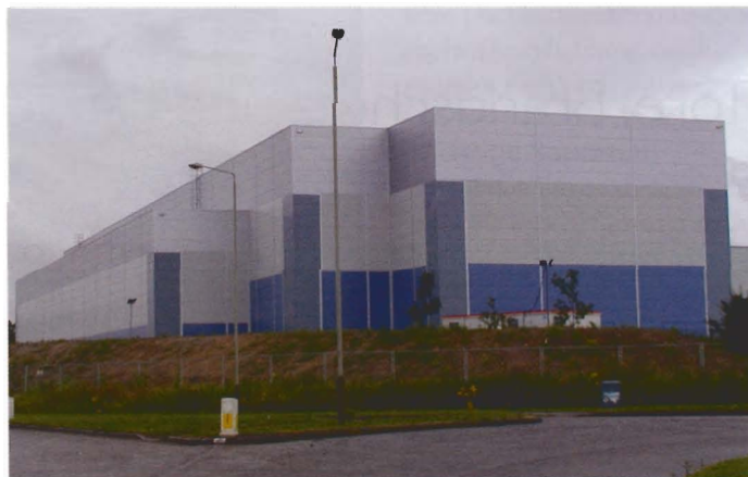
Walkers Snack Food Hochregallager. Bilder: Hammersen Elementbau
